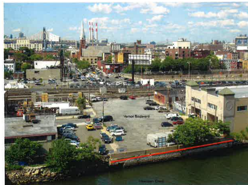
Vernon Boulevard Site from the GMDC Roof
