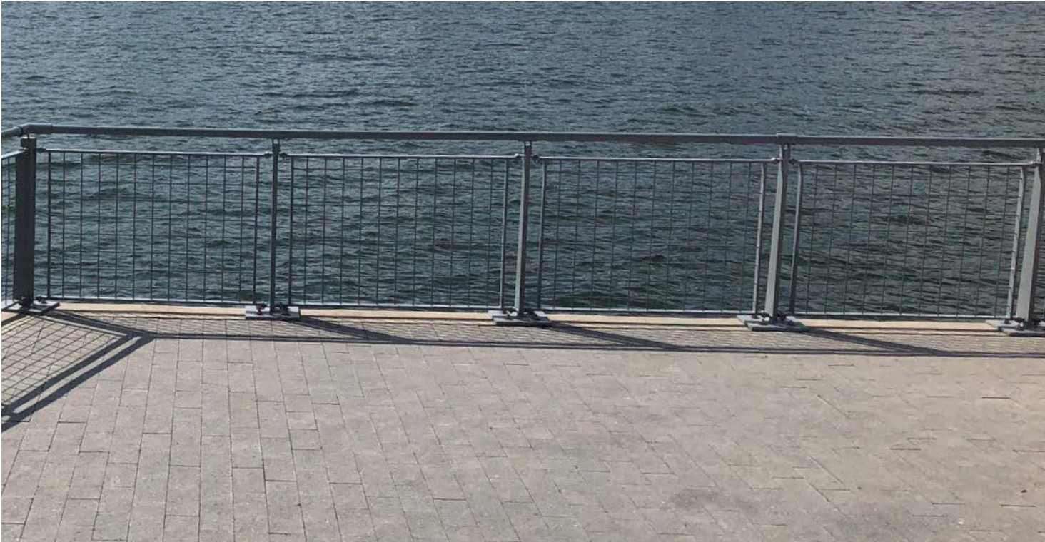
DCP STANDARD GUARDRAIL MAINTAINS VIEW TO NEWTOWN CREEK
