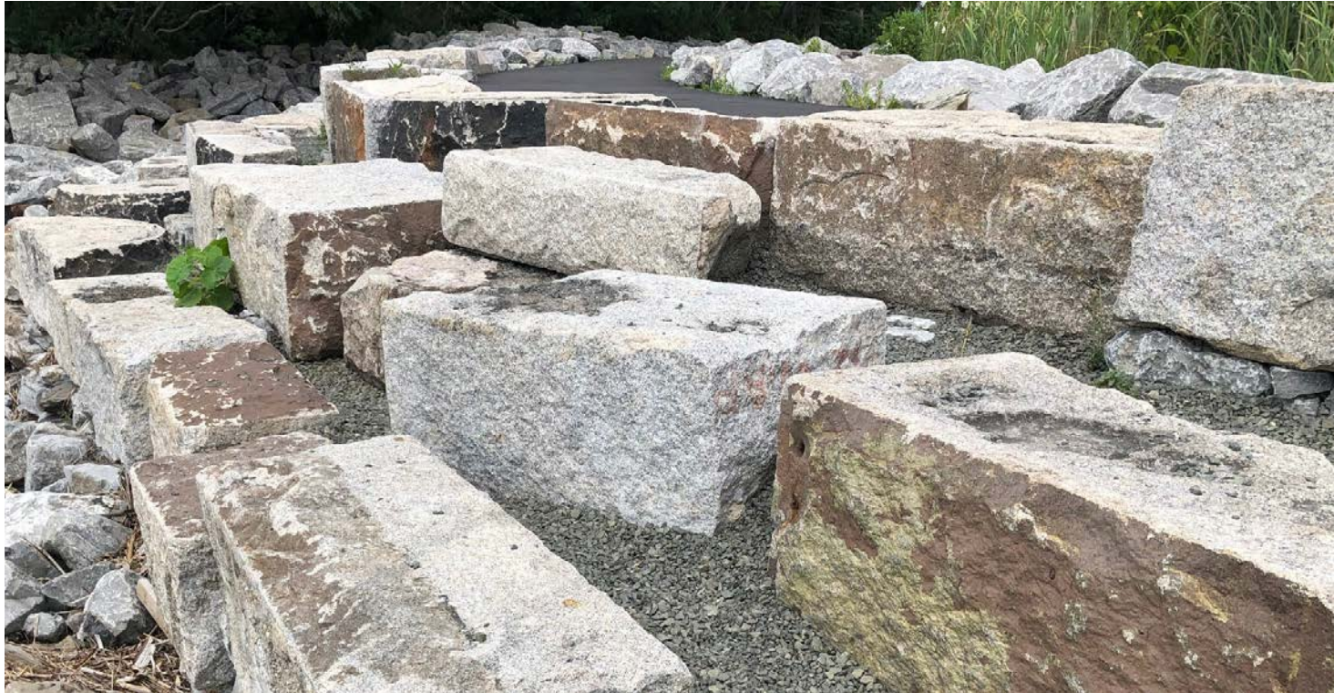
STACKED BOULDERS TO EASE TRANSITION TO ADJACENT, LOW BULKHEADS
